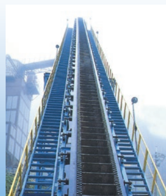
Crushed stone conveying
